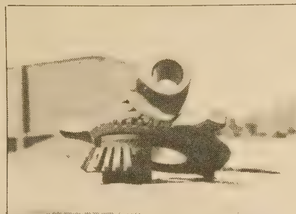
JACOBS CONNECTING GEAR WITH BLADE GEAR (NOTICE THE WEAR).
